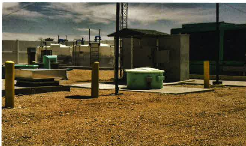
Big Dry Creek Lift Station
