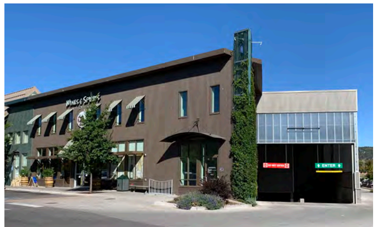
Screened loading area (Willits, Colorado)
