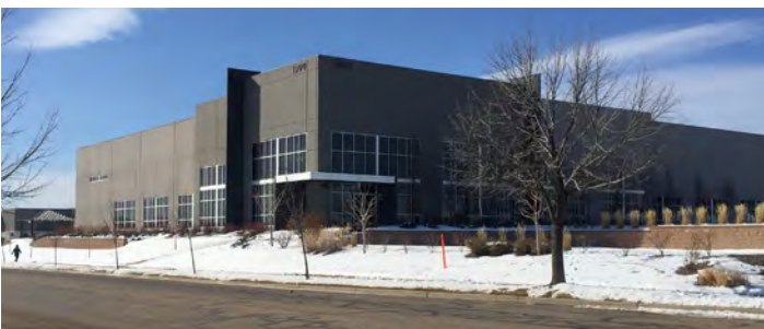
Screened parking at Colorado Tech Center (Louisville, Colorado)
