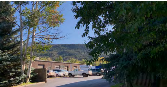
Screened loading area at Willits Design Center (Willits, CO)
