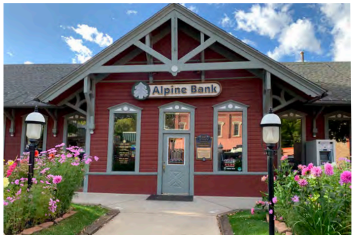
Local commercial use in a building that fits with neighborhood character (Basalt, Colorado)
