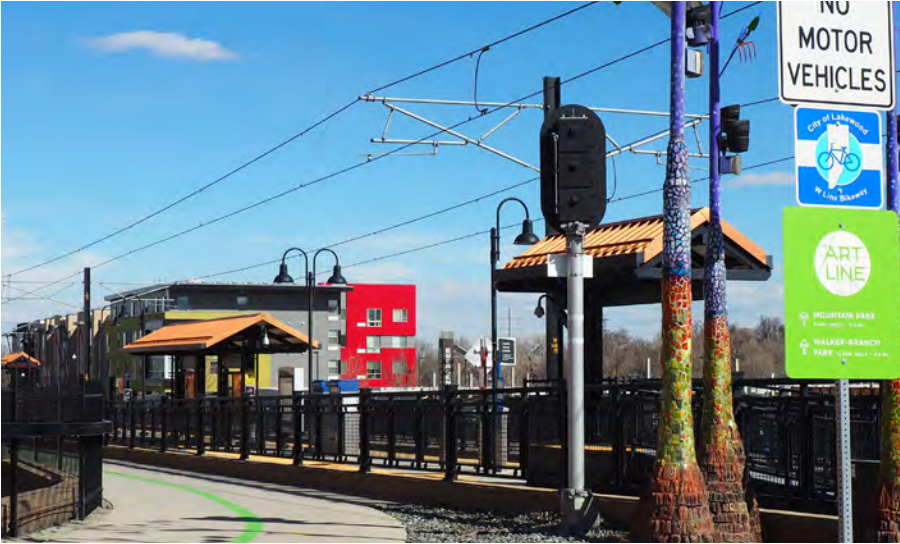
Transit-Oriented Development at Lamar Station Crossing along the 40 West Art Line and the W Light Rail Line (Lakewood, Colorado)
