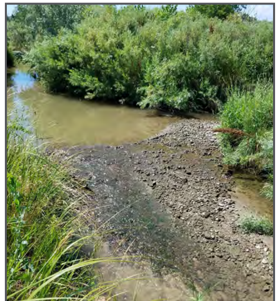
Failed grade control
