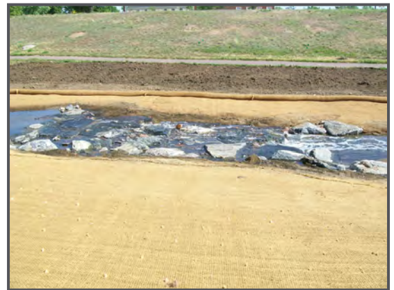
Riffle structure during construction with geotextile fabric along the banks
