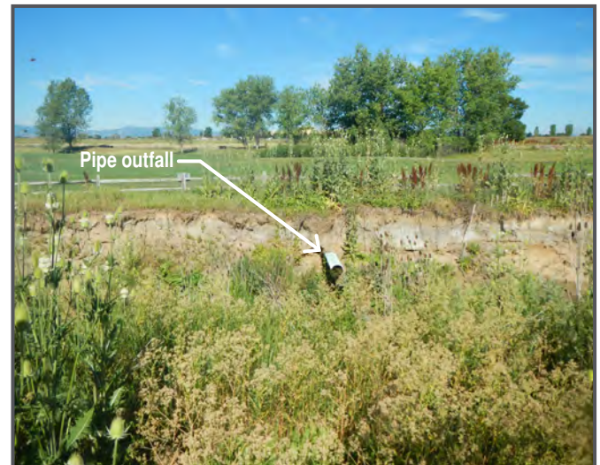
Bank erosion has caused this pipe outfall to be exposed with no protection
