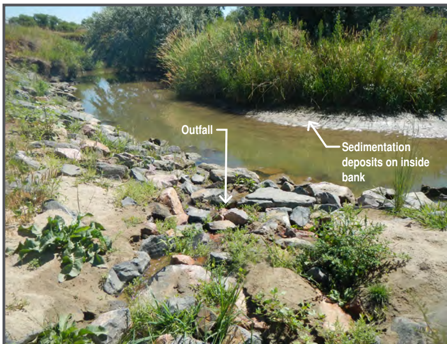
Although this outfall is stabilized with riprap, added vegetation will improve stability to the sides of the outfall
