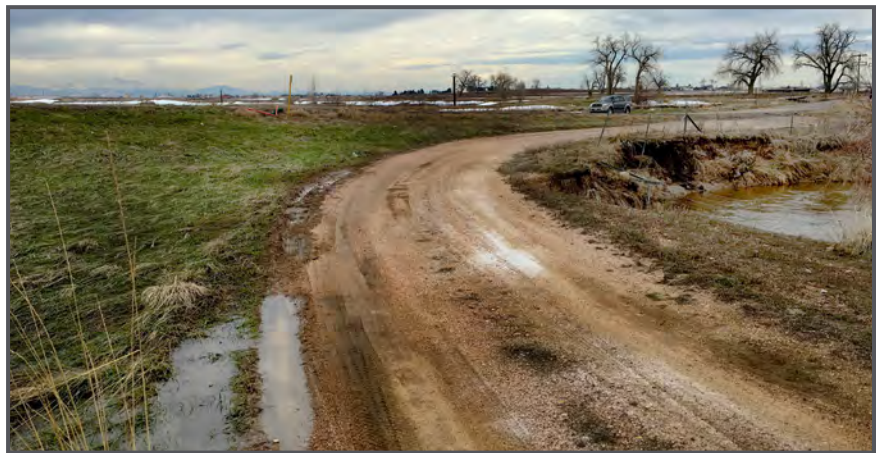
Big Dry Creek moving laterally into the oil/gas access road SW of Parcel VI
