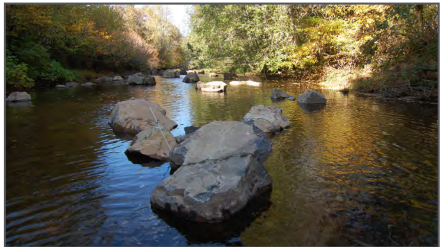
Boulder clusters installed
