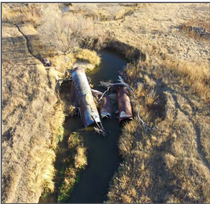
Failed culvert crossing within High Priority Reach 5 in Parcel III
