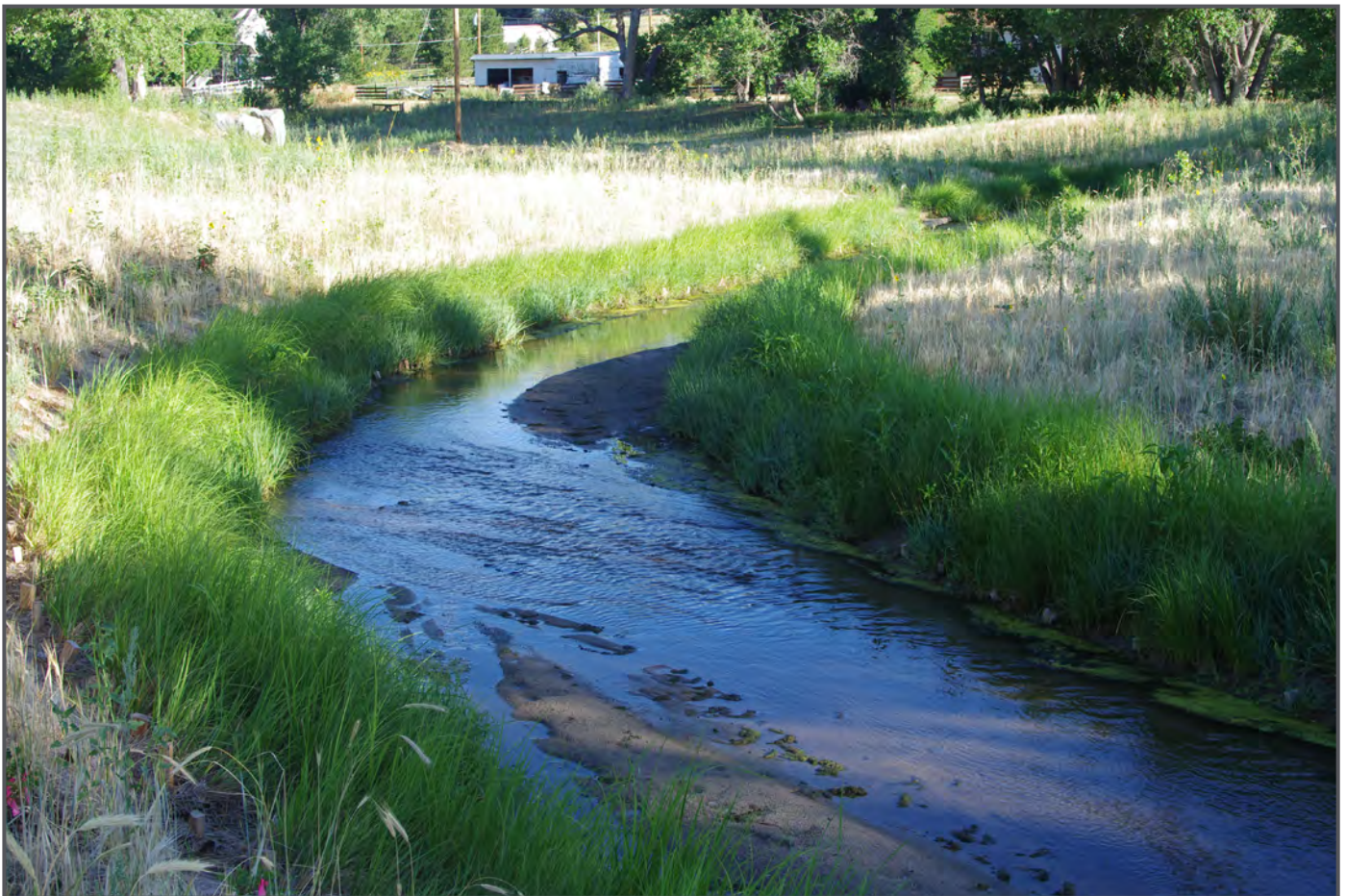
Wetland sod installed at the toe of the bank can provide immediate vegetative establishment for high priority areas
