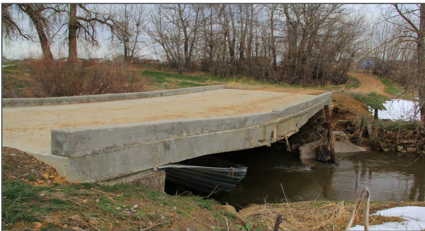
Corrugated metal hanging off of the bottom of the bridge at Small Project C
