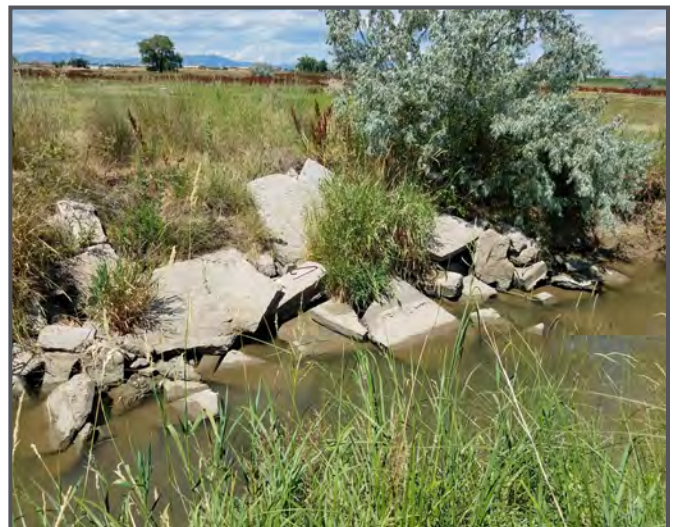
Eroding banks protected incorrectly with concrete scraps
