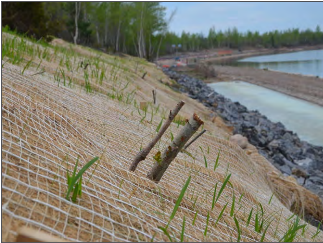
Geotextile bank stabilization used for revegetation
