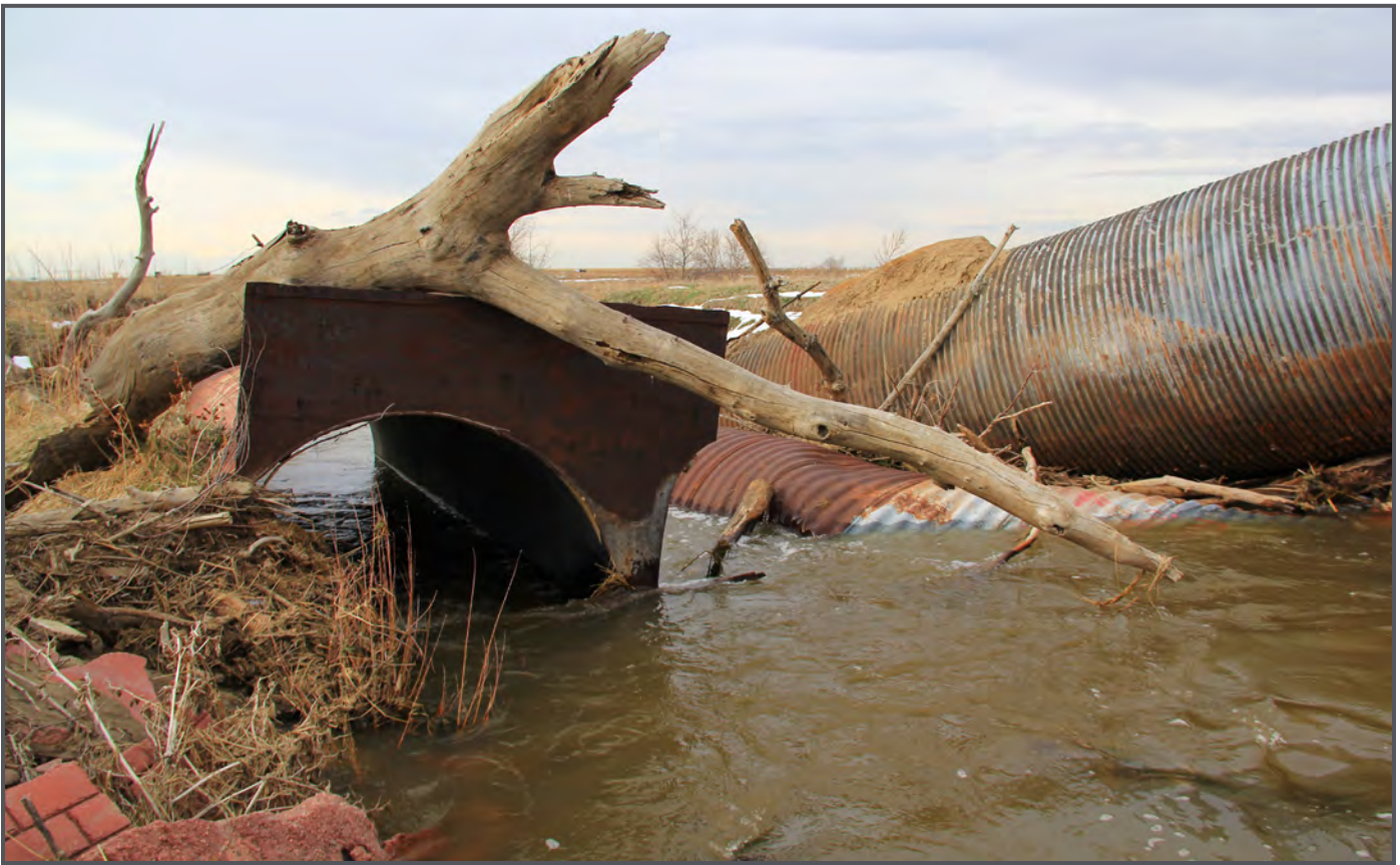
Small Project D contains blown out culverts that need to be removed from Big Dry Creek
