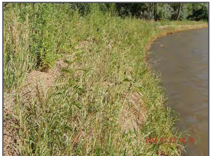
Willow stakes installed as part of a vegetated soil lift bank stabilization (after establishment)
