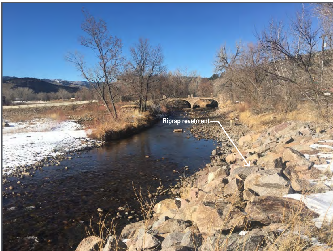
Example of a riprap revetment (armoring)
