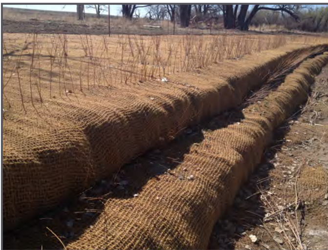
Willow stakes installed as part of a vegetated soil lift bank stabilization (at time of installation)
