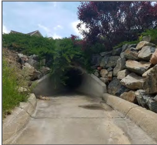
Concrete flared end section
