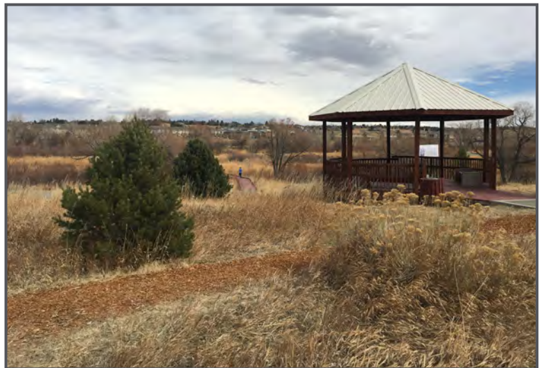
Elevated overlook using the grading of floodplain terraces to extend the overlook out over the floodplain
