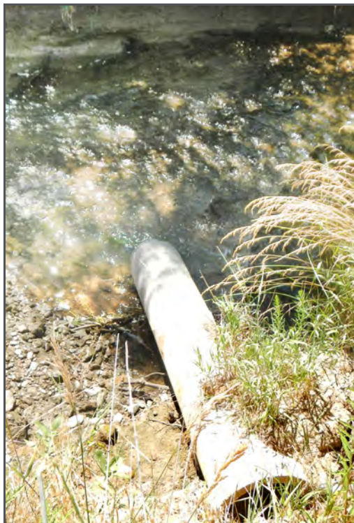
Pipe failure due to erosion on Big Dry Creek
