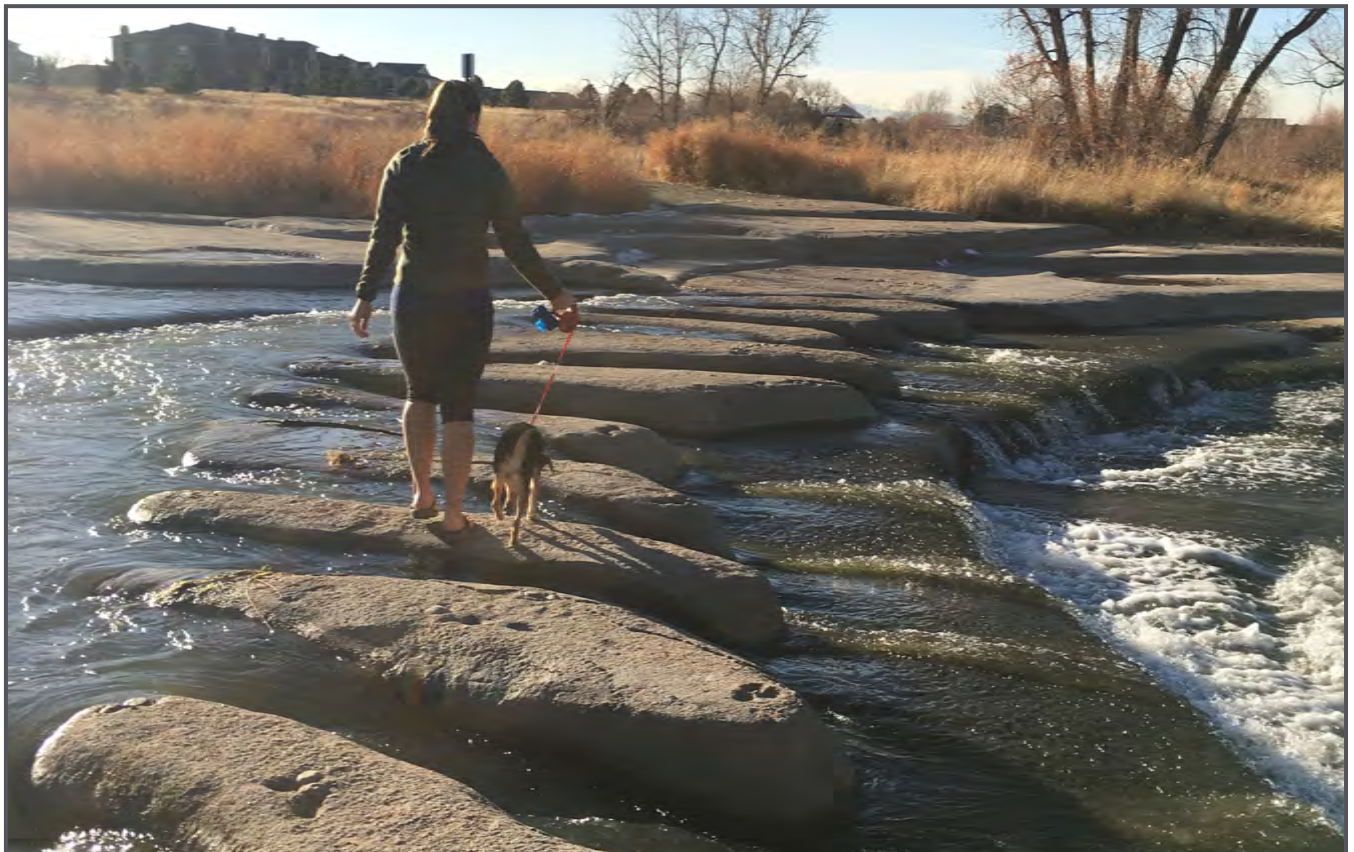
Example of a constructed drop structure that is also designed as a low-water crossing
