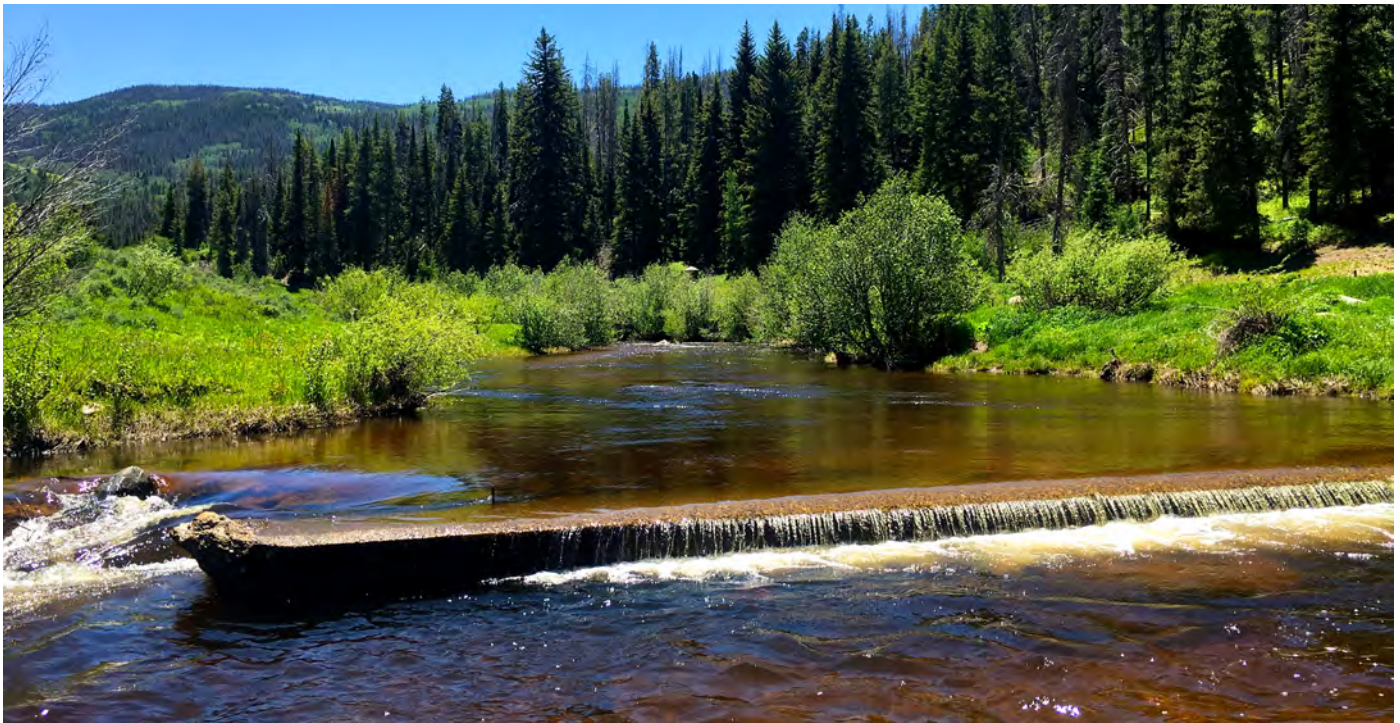
Example of an in-stream concrete sill
