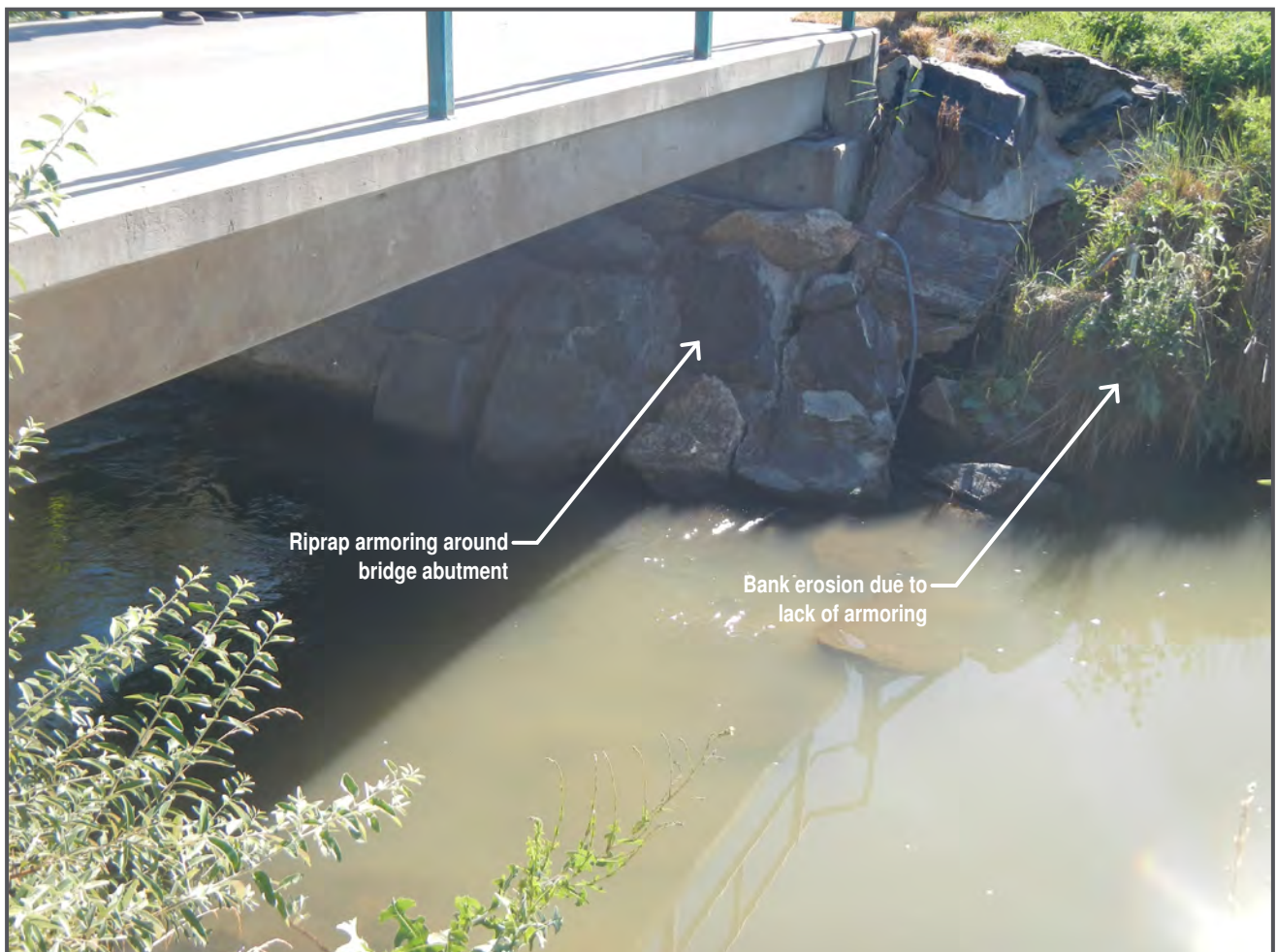
Abutments failing
