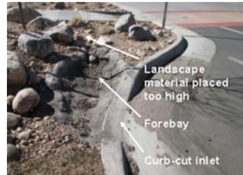
Not acceptable: Bioretention with curb-cut inlet. Landscape material (downstream of forebay) is placed too high and runoff cannot enter the BMP. Landscape material should be lowered about 3 inches below the inlet elevation
