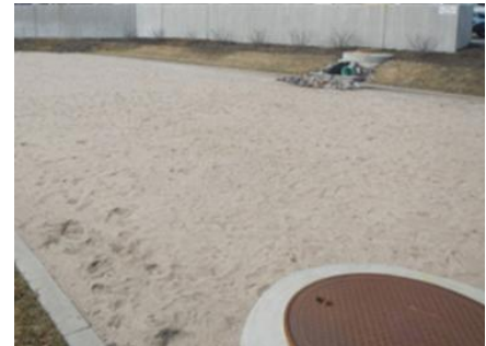
Acceptable: Typical sand filter
