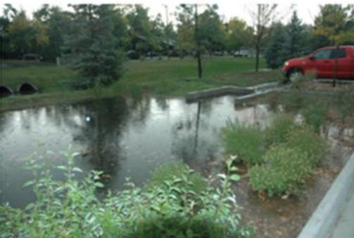
Acceptable: Typical bioretention with ponded runoff during rain event
