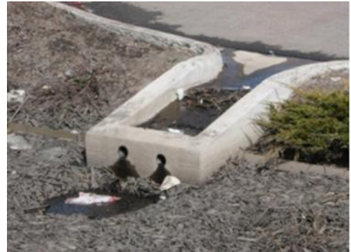
Not acceptable: Bioretention forebay that needs sediment and debris removed
