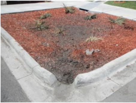
Not acceptable: Bioretention with uneven filter media grading. Maintenance is required to re-grade so that filter media is flat.
