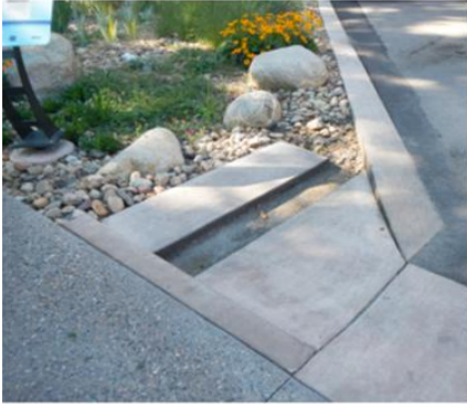
Acceptable: Bioretention forebay that has been properly cleaned
