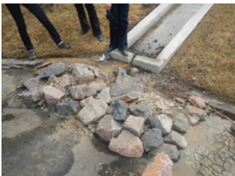
Not acceptable: Sand filter with rip-rap energy dissipater. Sediment that has accumulated near the rip-rap should be removed periodically. If maintenance of rip-rap is difficult, the owner may consider installing a forebay for easier maintenance.
