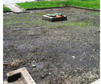
Not acceptable: Sand filter with obvious "cake layer" of sediment built up over time. This sand filter needs to be maintained by removing 1-2 inches of filter media and sediment throughout the entire BMP.
