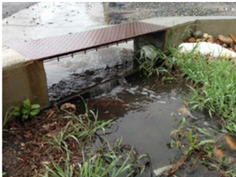
Acceptable: Bioretention with curb-cut inlet showing 3 inches of "fall" into BMP
