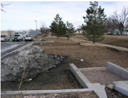
Not acceptable: Snow should not be stored on bioretention/sand filter BMPs
