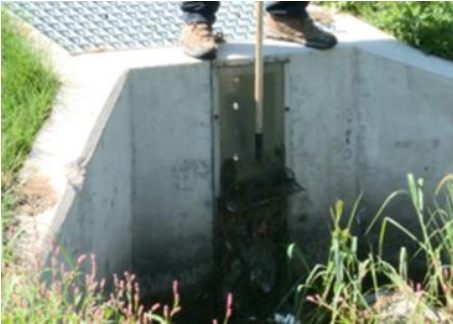
Acceptable: Cleaning the well screen gently using a garden rake
