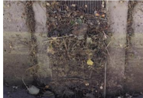
Not acceptable: Well screen that is clogged with debris. Maintenance is required to prevent standing water.
