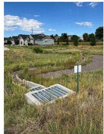
Ideal vegetative coverage and length in a detention basin
