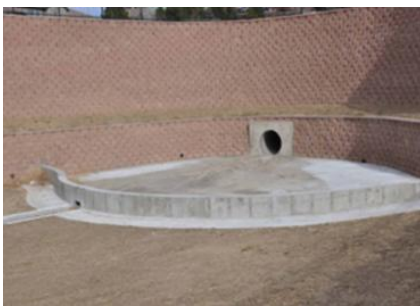
Acceptable: Clean forebay in working condition after recent maintenance. A small amount of sediment is noticeable from a recent storm, but there is no trash or other debris present.
