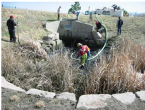
Acceptable: Using a vacuum truck to remove sediment from the micropool
