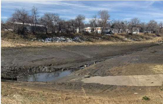
Not acceptable: Vegetative die off due to drowning from a plugged system.
