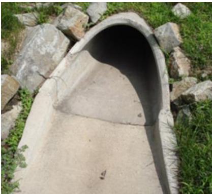
Acceptable: Clean inlet after proper maintenance
