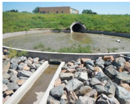
Not acceptable: Forebay with excess sediment that needs to be removed. Vegetation growing in the forebay is a typical sign that maintenance is needed.
