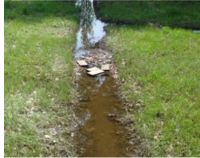
Not acceptable: Trickle channel that needs maintenance. Standing water in the trickle channel is a sign that sediment and other debris are blocking the flow of water.
