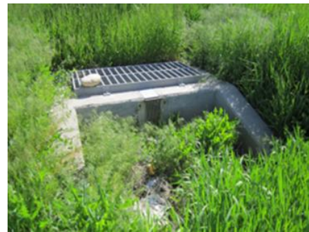
Not acceptable: Sediment, debris and vegetation built up in front of outlet structure
