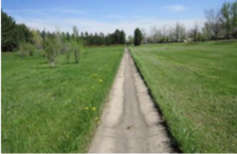
Acceptable: Clean trickle channel with no sediment, debris, or woody vegetation nearby
