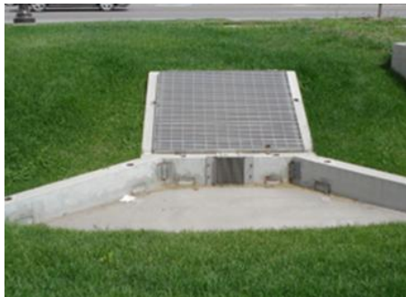
Acceptable: Picture of a well-maintained outlet structure
