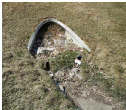
Not acceptable: Inlet with sediment, trash and other debris that needs to be removed.
