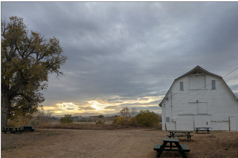
The Rietzenstein Barn within the Big Dry Creek Open Space was constructed in 1923 and has been well preserved.
